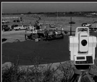
3-D Profiler System Utilised in multi-sloped concrete paving
