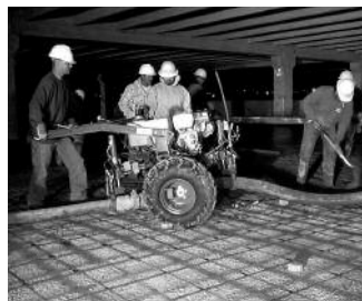
HoseHog Drags concrete hose
