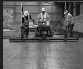
CopperHead XD 3.0 Utilising laser technology in a walk behind unit
