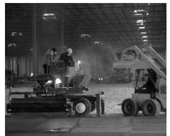
STS-132 Topping Spreader
